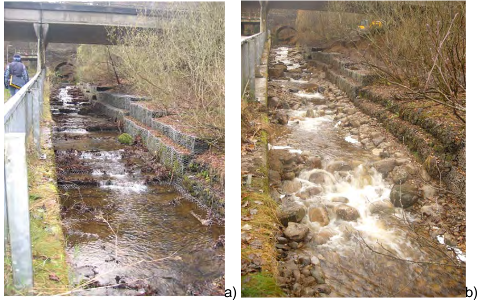
Figure 10.5 Case study of boulder placement restoration. a) before restoration activities, b) after boulder placement (from RRC).
