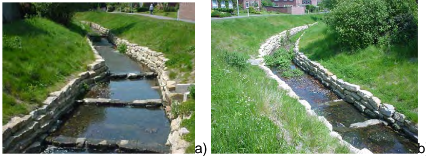
Figure 10.1 Photos of step-weir placement a)looking upstream, b)looking downstream.
