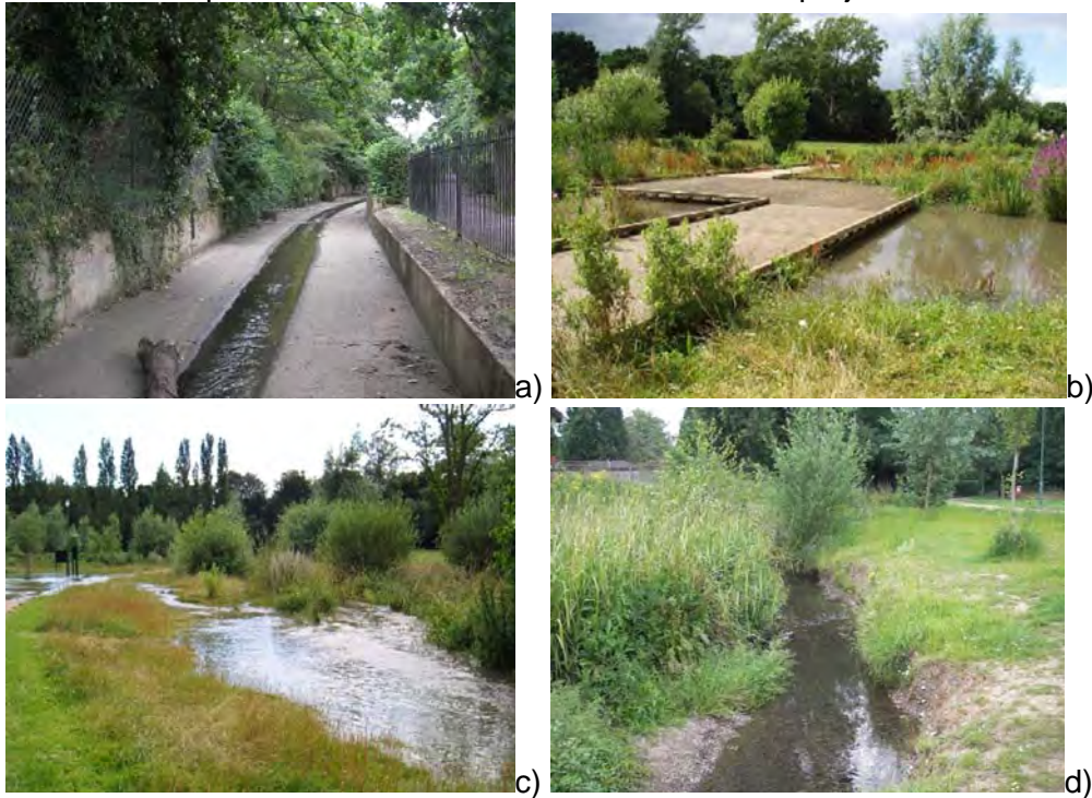
Figure 10.5 Process of repositioning a concrete lined channel into a new riverbed, showing a) original concrete-lined channel, b) floodplain features in newly created channel, c) new channel floodplain connection, d) new channel cut through park.
