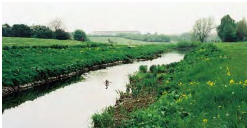
Figure 10.3 River Skerne after river narrowing with type-A vegetation ledges (from RRC river restoration manual).
