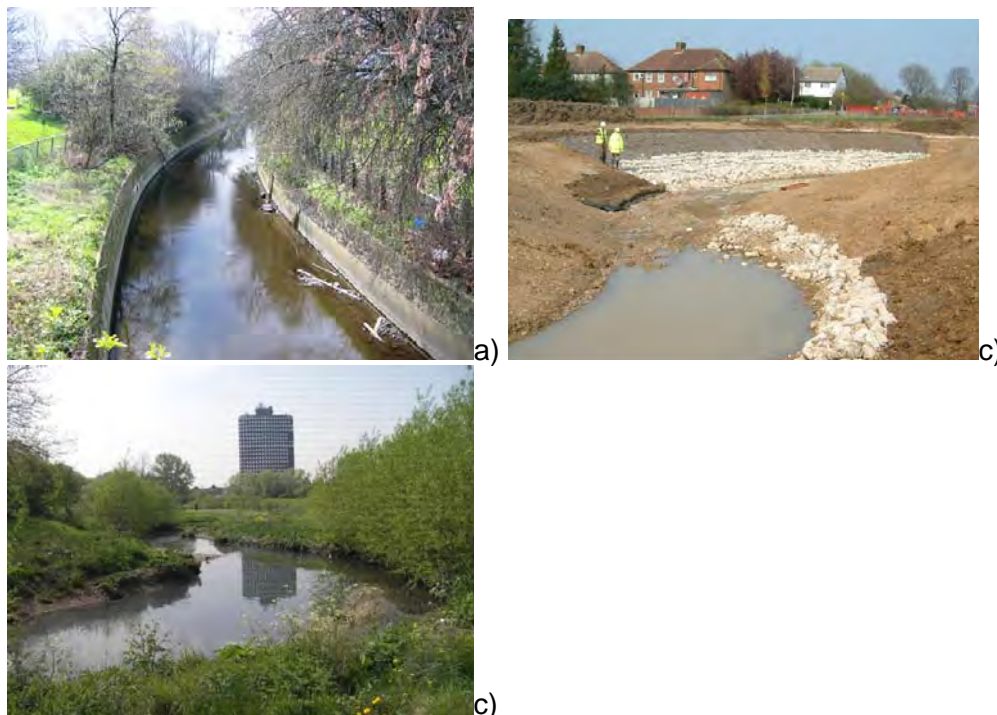
Figure 10.4 Images from hard bank removal on the River Trent in London. a) concrete-lined channel before restoration, b) construction of riverbed and banks after concrete removal, c) natural vegetation and bank features.
