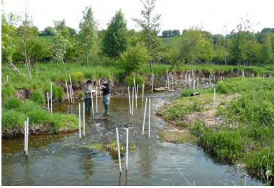
Figure 8.1 Network of mini-piezometers (PVC tubes) installed to monitor VHGs and seepage fluxes in the river (photo: Daniel Käser).
